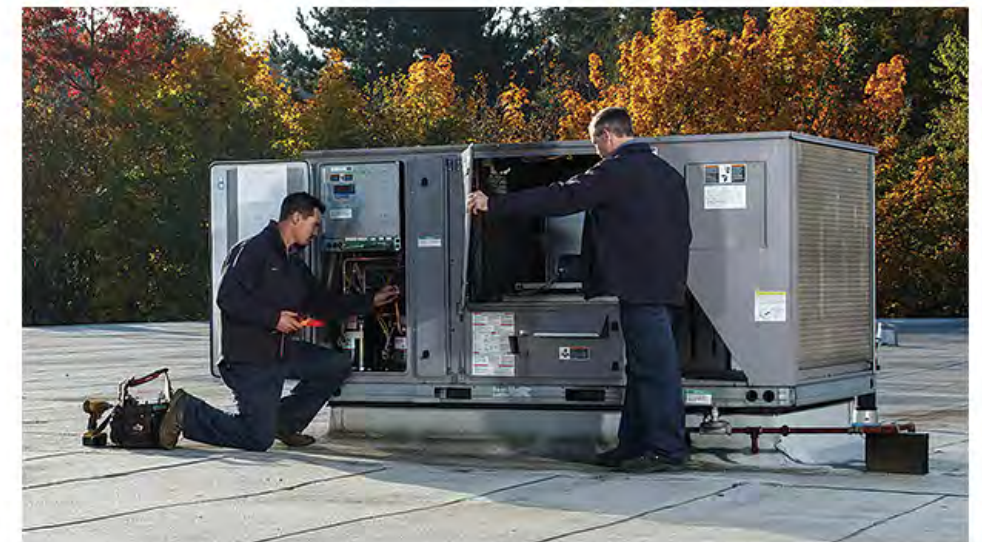
Reitmeier employees Devon Brown, service technician, and Michael Taal, senior service technician, work on a rooftop unit.
